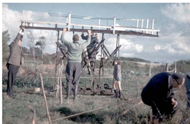
Figure 12b. Another photo of Patrick and Frank Hyde assembling a radio antenna at Henry Brinton's Selsey home in 1961. Patrick is still on the left, and Frank is still up the ladder. From Patrick's personal photo archive.
